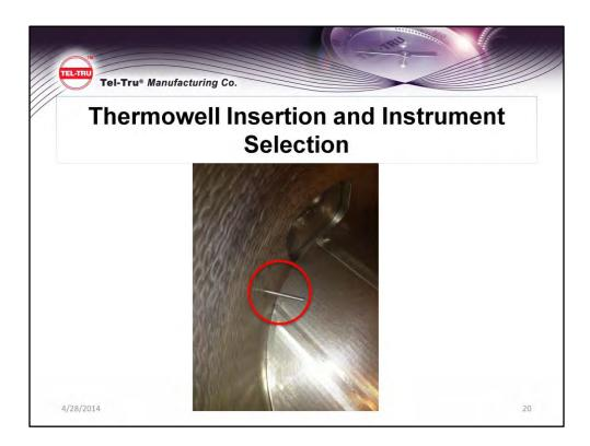
Image shows a thermowell shank inside a mash tank. This portion of the thermowell is called the insertion length. Be sure to consider the ideal location and position for your Thermowell before installation. You also want to ensure that there are no moving parts inside the tank that will come in contact with the well.
